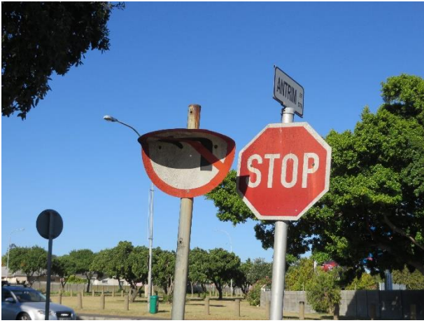
Figure 35 Bent and disorientated signage
