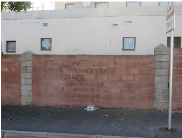
Figure 22 Graffiti on a building
