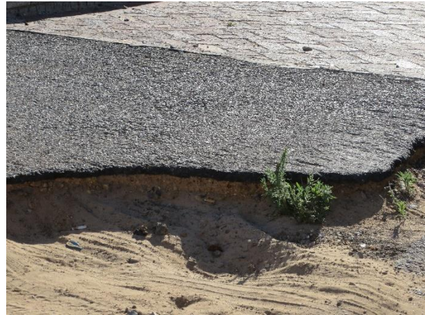
Figure 40 Poor sidewalk surface
