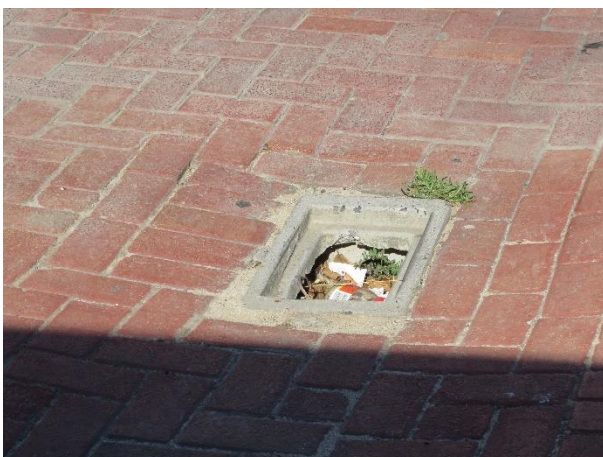
Figure 43 Open manhole on sidewalk
