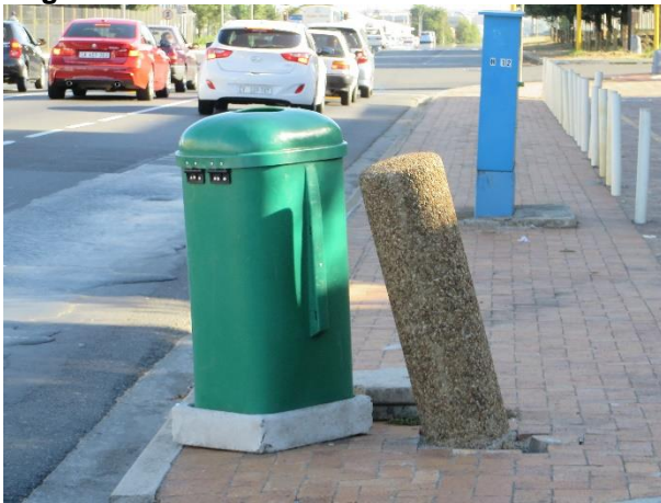
Figure 41 Damaged public infrastructure
