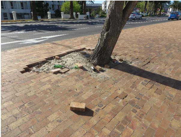
Figure 39 Poor sidewalks in isolated locations
