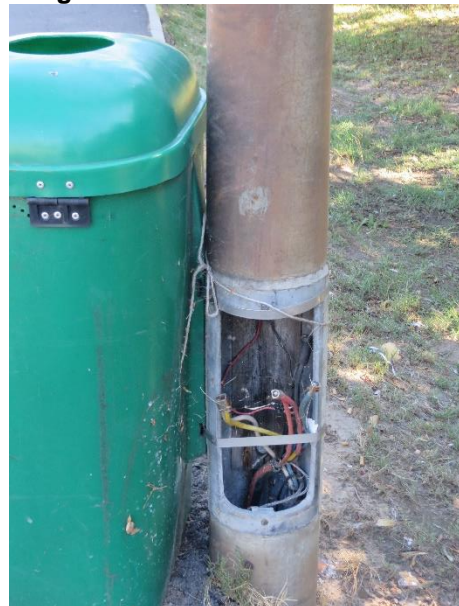
Figure 42 Street light poles with no electrical covers
