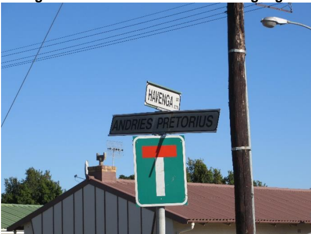
Figure 37 Bent and disorientated signage
