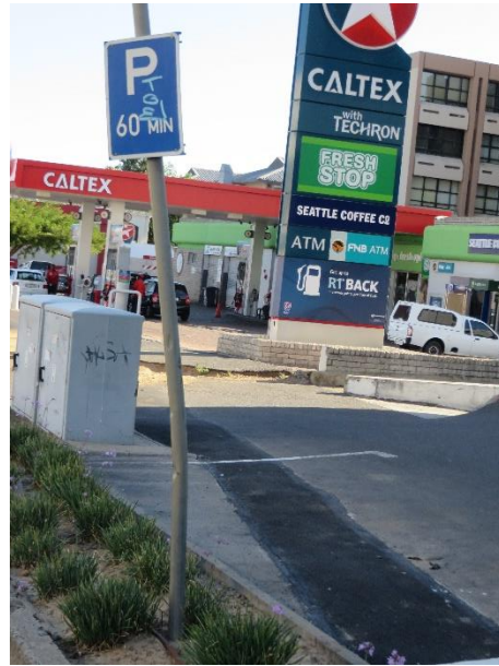
Figure 36 Bent and disorientated signage
