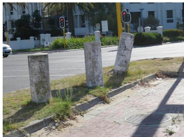
Figure 44 Damaged public infrastructure
